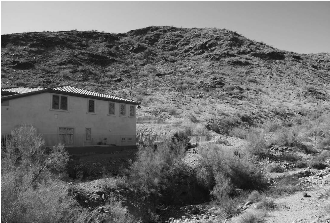
Fig. 1. A home built in 2006 and 2007 in a suburban neighborhood of Phoenix, AZ., directly on the depositional area of debris flows. Although the slope catchment area is <10,000 \text{ m}^2 , at least five distinctive sets of debris-flow levees occur immediately above this home, with no structures above the home to divert future debris flows.
