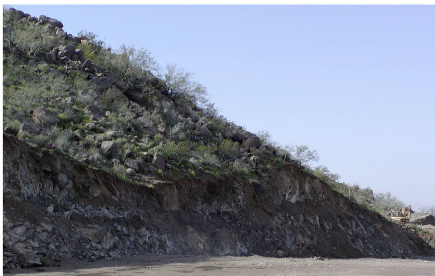
Fig. 1. Construction at the Las Sendas subdivision in the Utery Mountains of Mesa, Arizona, exposed hundreds of meters of granodiorite bedrock. These cross-sections of inselbergs made it possible to examine 300 fractures hosting fills of eolian dust and rock fragments. After opening fractures with a rock hammer, fines were washed away and data tabulated on the presence of orange iron films, the presence of an outer band of black rock varnish, and the presence of HCl-reacting laminar calcrete.
