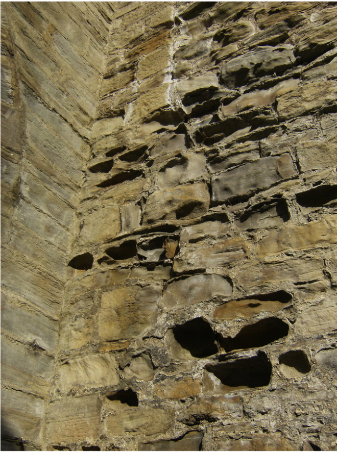
Fig. 9. Tafoni formation on the outside walls of Durham Cathedral, UK (Photo: Lisa Mol).
