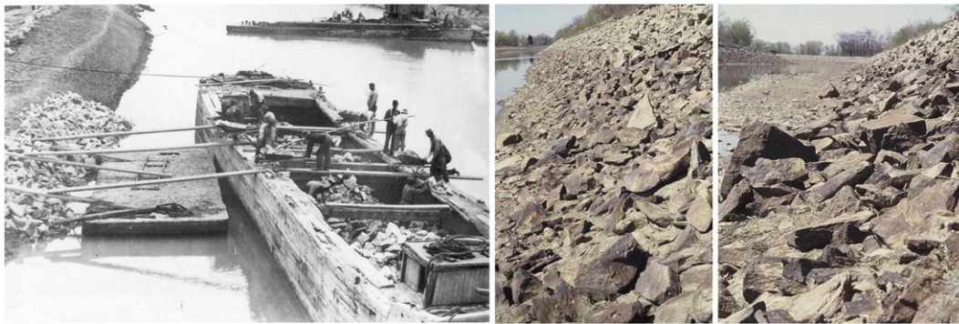
Fig. 3. Historic photograph of boulders quarried in 1913 being placed along the Erie Canal, with a view of the boulders a century later. Rock varnish forms in the area experiencing periodic inundation and also in subaerial settings that do not experience splash. The sample analyzed here derived from a subaerial setting.
