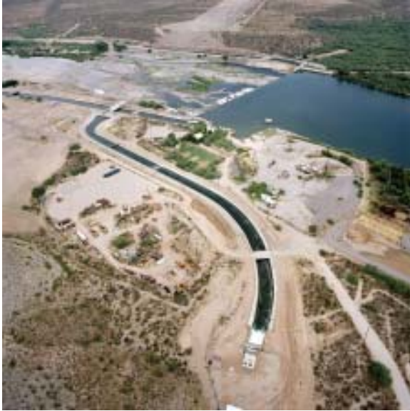
Figure 6.1 Granite Reef Diversion Dam.
