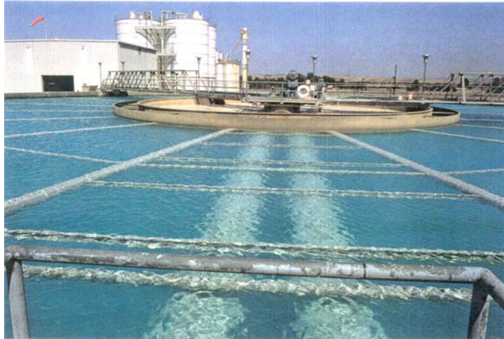
Figure 3.8 Solids Contact Reactor at the Yuma Desalting Plant.
