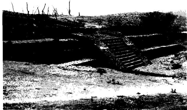
Figure 2. Photograph of the west (front) façade of the Yautepec palace.
