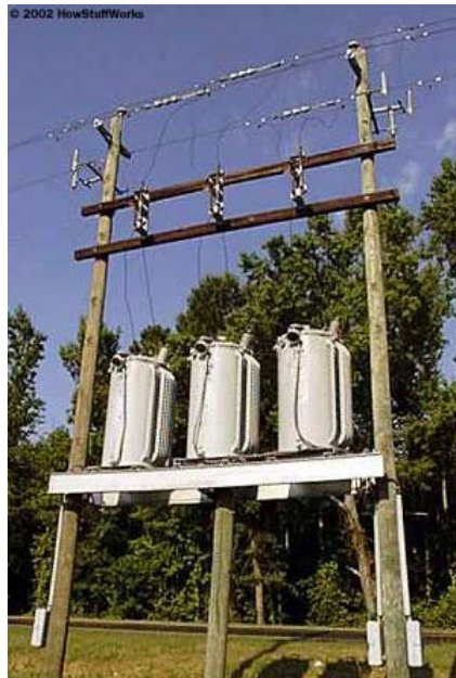
A typical regulator bank
