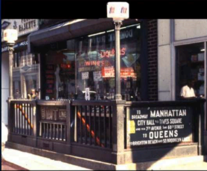
Entrance to Lawrence Street Station 1969
