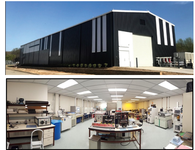
The National Center for Reliable Electric Power Transmission (NCREPT)
