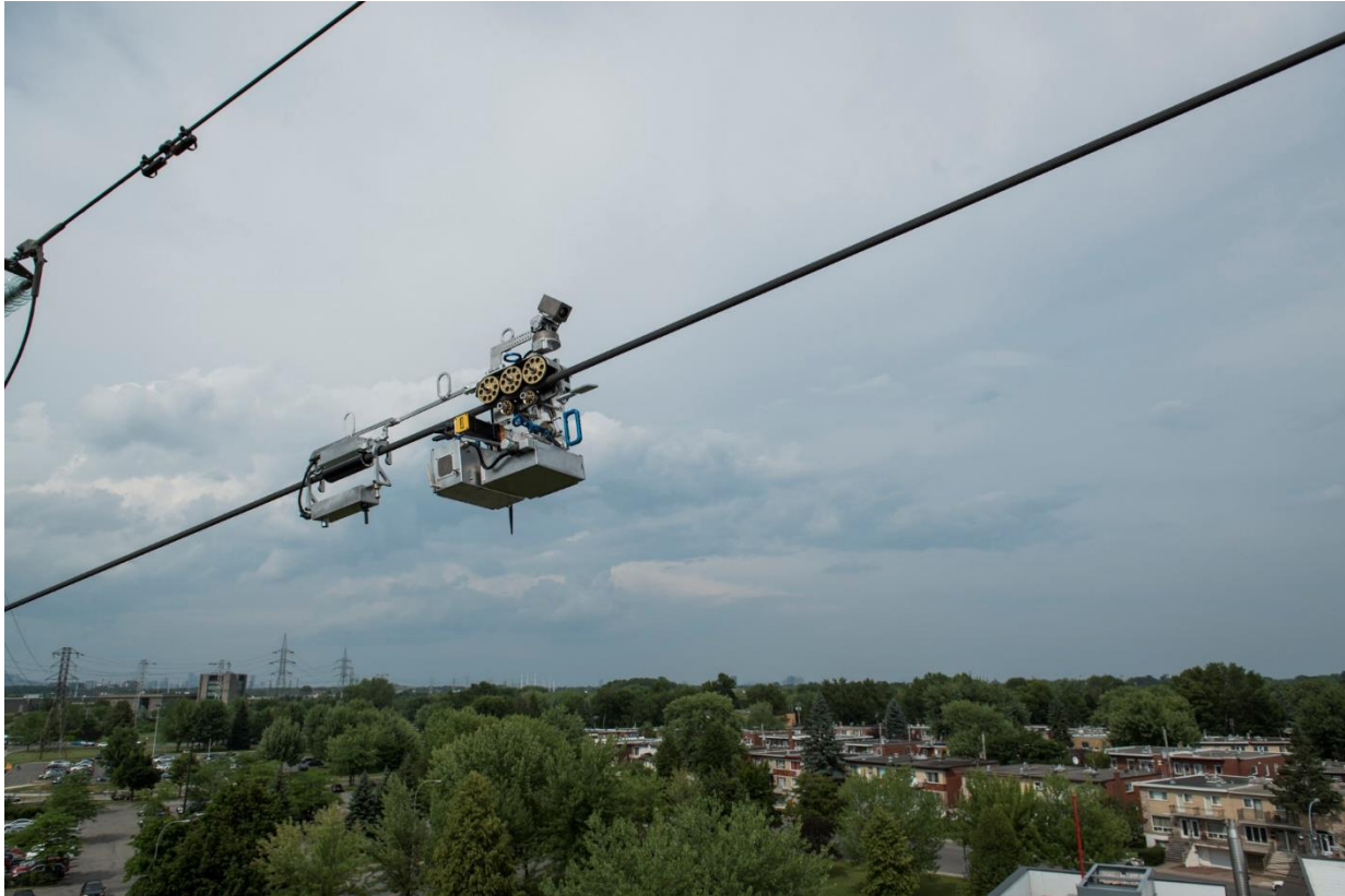
The LineRover remote-controlled robot (right), by MIR Innovation, a subsidiary of Hydro-Québec, tows the LineCore sensor during a conductor inspection. Photo credit: Hydro-Québec
