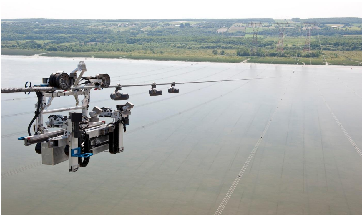
The LineScout, by MIR Innovation, a subsidiary of Hydro-Québec, inspects a ground wire and 735-kV lines near Ile d'Orléans in the Saint Lawrence River, east of downtown Québec City, Québec, Canada. Photo credit: Hydro-Québec
