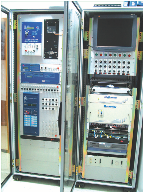
figure 6. Substation automation training simulator.
